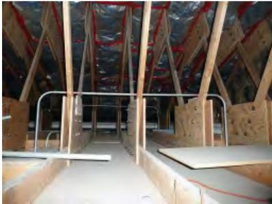
Attic with R-19 at roof underside
